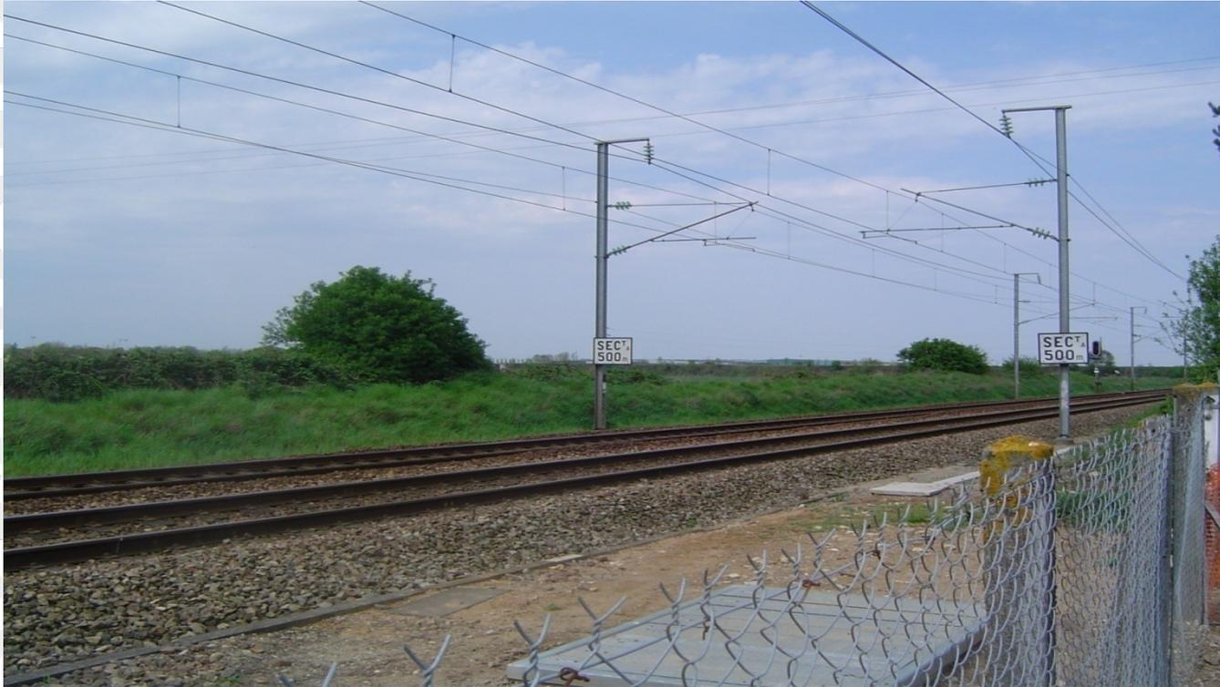
catenary : system of overhead wires used to supply electricity to the locomotive equipped with a pantograph
